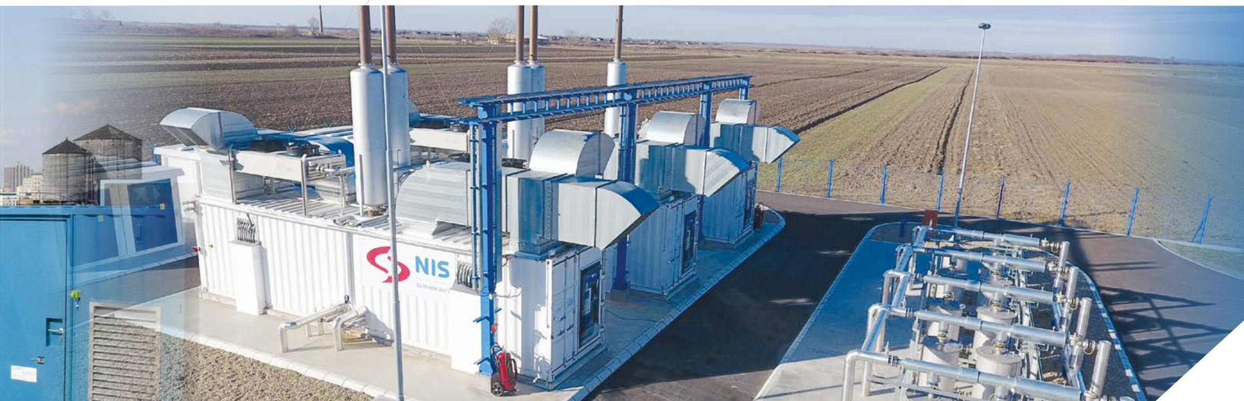
// 5 x 400 kW CHP with emergency operation functionality for an office building in Manhattan, USA
